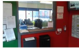
Glass panel partition to transport office
