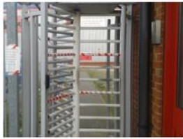
Regular cleaning of turnstile
