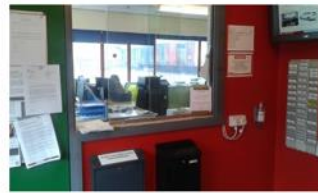
Glass panel partition to transport office
